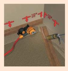
To join two mouldings that are positioned along the same wall, you can cut them at right angles. However, a scarf joint is recommended. Position both baseboards as they will be on the wall and cut them at the same 45 degree angle. Please note that the baseboard must be cut at right angles when used as a door frame.
